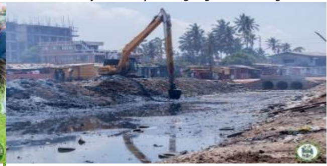
Ongoing desilting of drains in Accra
