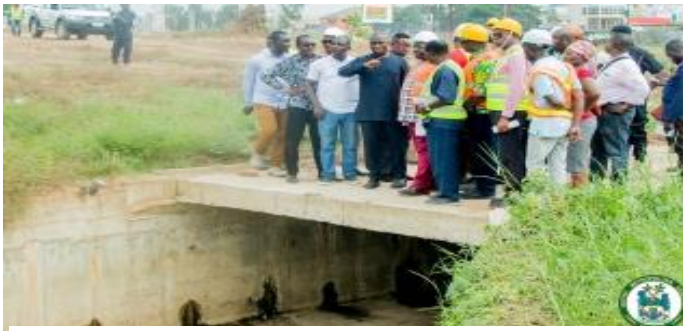
Work begins on underground drain at Kaneshie First Light to prevent constant flooding
