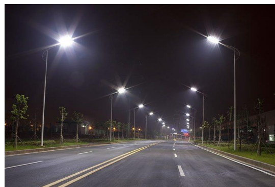
View of Assembly Street lighting project
